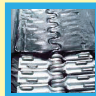
Clip joint sealing
